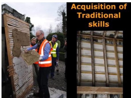
On-site training for the farmer in use of lime mortar as a traditional plastering technique (Heritage Council)
