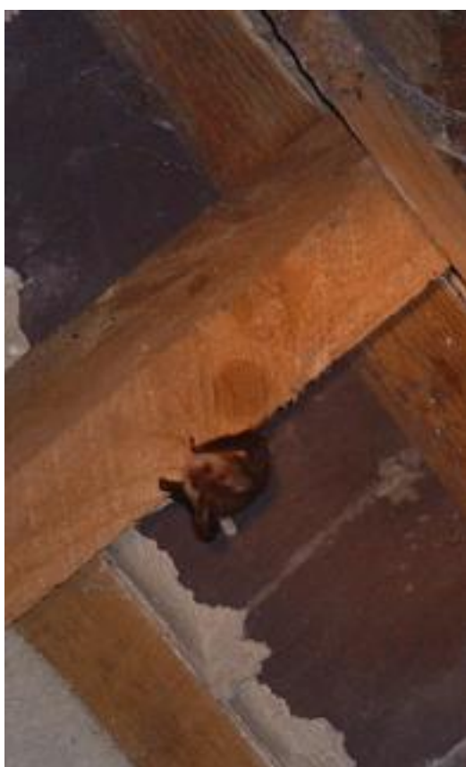
Brown long eared bat resting on a rafter (Heritage Council)
