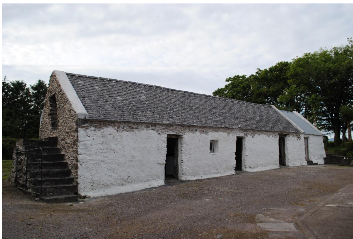
Traditional farm building in Co. Kerry after restoration works. (Heritage Council)
