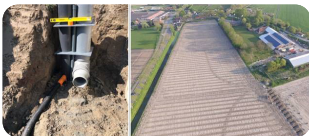
Evacuating water © Novifarm
