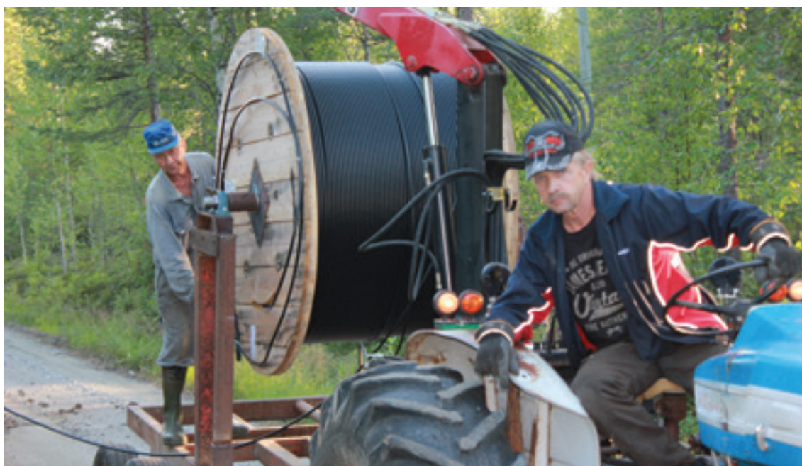
© Village Optical Fibre Network Cooperative of North-Western Kuhmo
