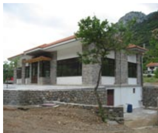
Picture 9: Greece — Construction and equipping of a tavern
