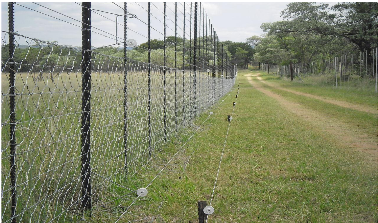
Figure 5: electric fencing with reinforced wire mesh at the base (Source: https://chemvet.co.za/ )
