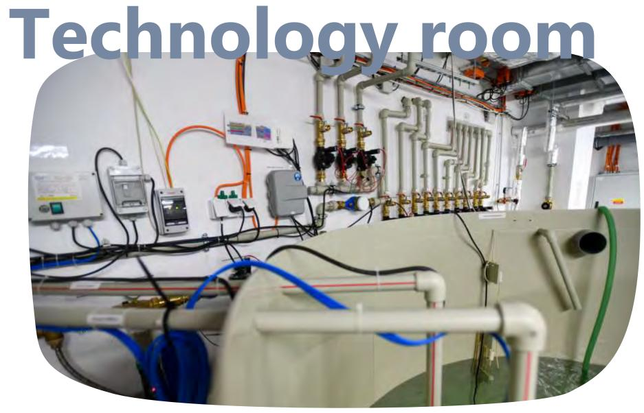
Technology room consist of grey water treatment system with a capacity of 1500l/day, the purified water undergoes hygienic treatment (UV lamp and chlorination) and then goes to the root filter. A water storage tanks for irrigation, water is pumped from there to the roof (3 circuits) and to the facade (9 circuits). The water for irrigation of the facade is fertilised. And separate pumping station for flushing toilets.
