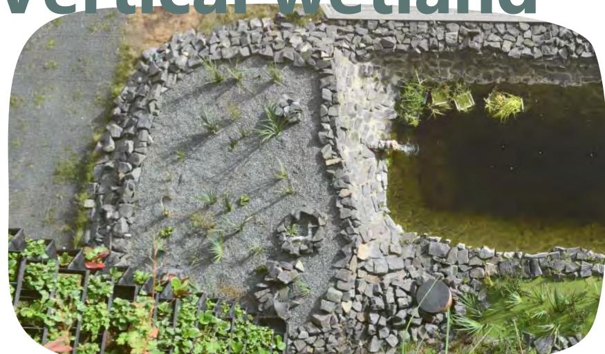
The vertical flow wetland is a natural tank composed of aggregate, which is planted with wetland vegetation (Kyprej willow, Yellow Iris, and Marsh Fescue). Functionally, it is an unheated aerobic biofilter, with a total area of 20 m<sup>2</sup> and a usable volume of 13.5 m<sup>3</sup> divided into two parts with different functions.
