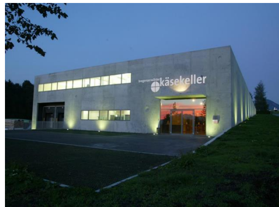
Figure 3.2: The Bregenzerwald cheese cellar is the heart of the organisation and the administrative headquarter; Source : https://www.kaesestrasse.at/
