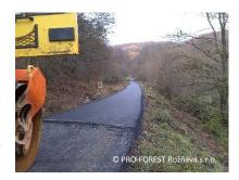
Construction works included modifying the adjacent slopes, constructing sluices including concrete fronts from the reinforced concrete pipes, as well as concrete drainage channels, drainage ribs, road ditches and drainage gutters. A wooden lookout tower was also constructed.
