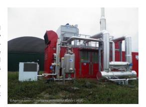
More specifically, using livestock manure and wastewater from the milking room and the milk processing unit, the system produces sufficient electricity and heat to operate the farm and the processing unit.
