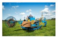
Submerged drainage is an effective measure to slow soil subsidence and this project supports a large-scale construction of such a system. The project also aims to widely share the knowledge gained. Thus, it is piloting an approach that could be applied in other comparable peat meadow areas.
