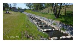
In order to allow fish to cross the stream once again, two new fish ladders were constructed. The pond in the monastery park was revitalised. Finally, a flood channel with an automatic weir was built to ensure flood runoff.
