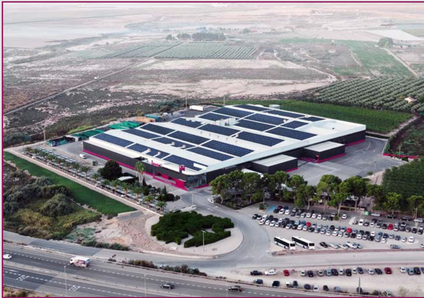
Photovoltaic solar panels
